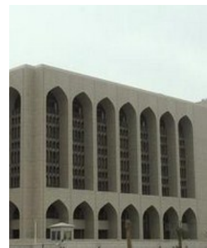
The United Arab Emirates central bank said it was making it easier for Islamic banks to access its special lending facility by expanding the range of collateral they can use.
